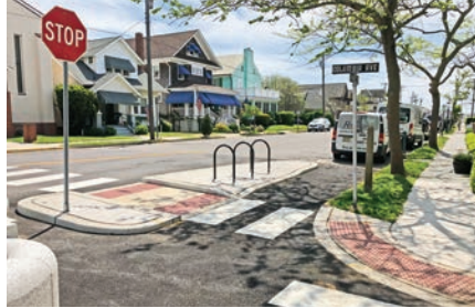
Road Diet, Bulb-Outs, Curb Ramps and more Cape May, New Jersey
