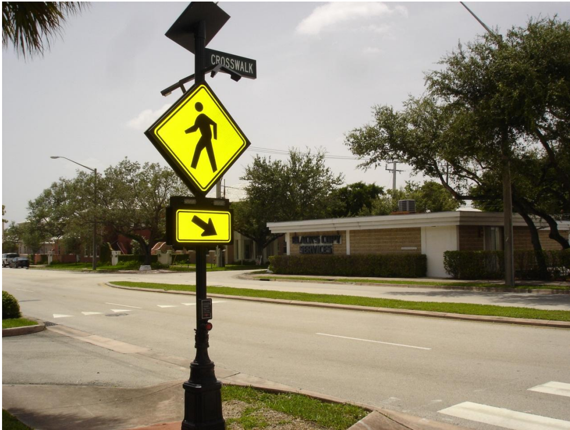
Pedestrian warning sign (W11-2) at a high emphasis crosswalk. Note the yield bars (series of isosceles triangles painted on the approach to the crosswalk). (Credit: Kimley-Horn and Associates, Inc.)
