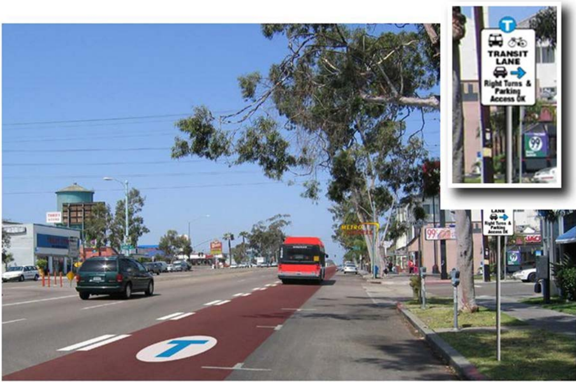
Simulation of a shared bus and bike lane adjacent to on-street parking (Source: San Diego Association of Governments)
