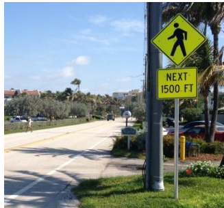
Advance pedestrian warning sign with distance plaque (Credit: Kimley-Horn and Associates, Inc.)
