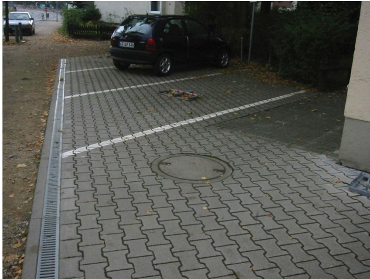
Permeable paving and a trench drain in a parking area (Credit: Stephanie Landregan)
