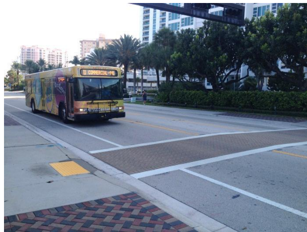
Controlled mid-block pedestrian crossing; note traffic signal structure overhead (Credit: Kimley-Horn and Associates, Inc.)
