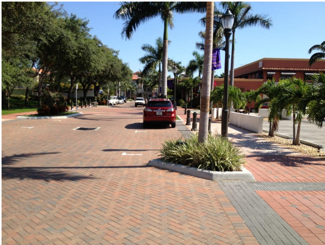
Landscaped curb islands, decorative pavers, and no centerline stripe help give this festival street a sense of place while calming traffic (Credit: Kimley-Horn and Associates, Inc.)
