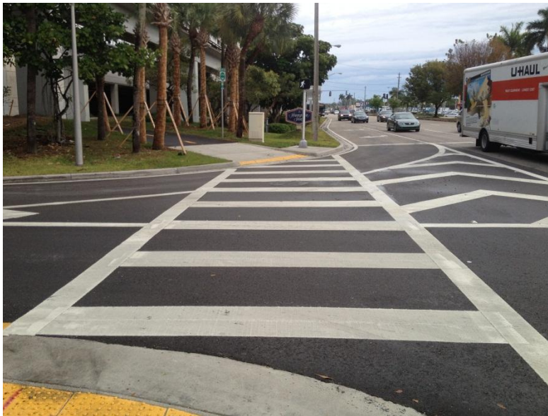
FDOT special emphasis crosswalk; note this design may have been improved by a channelization island for refuge (Credit: Kimley-Horn and Associates, Inc.)
