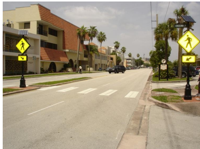
Rectangular rapid flashing beacon (RRFB) crossing safety device with median refuge (Credit: Kimley-Horn and Associates, Inc.)
