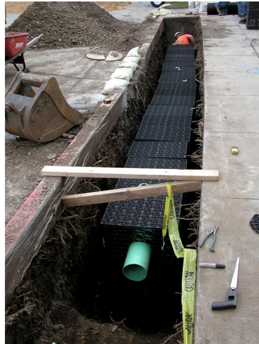
Infiltration trench with perforated pipe during installation (Credit: Neil Shapiro)
