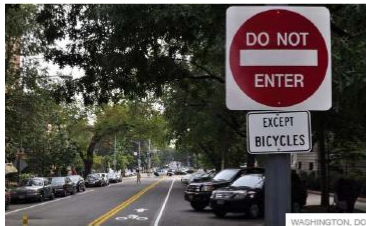
Contra-flow bike lane (Source: NACTO Urban Bikeway Design Guide)
