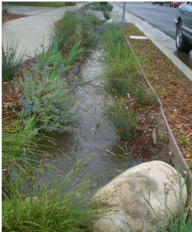
Sidewalk-adjacent swale during storm event
