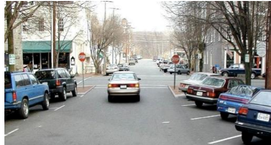
Example of curb extensions (Credit: Marcel Schmaedick)
