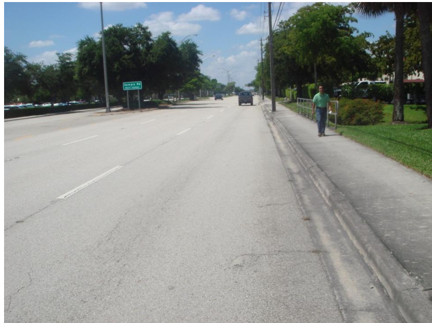
High automobile level of service, but poor multi-modal level of service (Credit: Kimley-Horn and Associates, Inc.)
