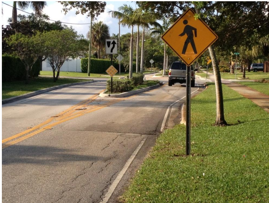
Short median adjacent to uncontrolled intersection (Credit: Kimley-Horn and Associates, Inc.)
