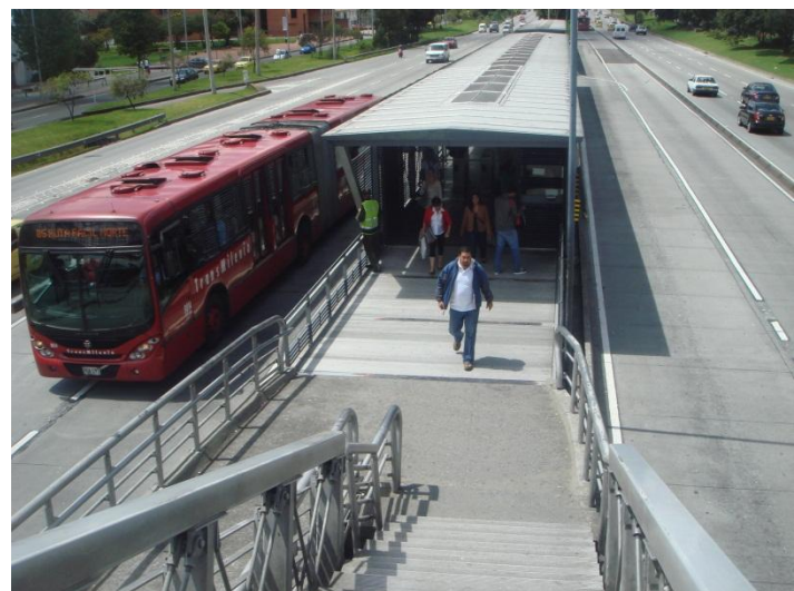
Busway in median with center platform stations: TransMilenio BRT, Bogotá, Colombia (Credit: Stewart Robertson)
