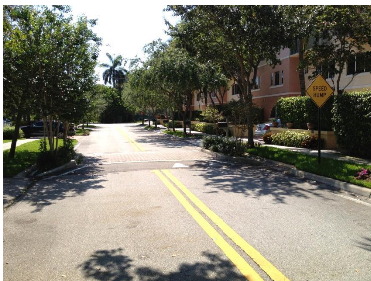
Speed table and lane narrowing with warning sign (Credit: Kimley-Horn and Associates, Inc.)
