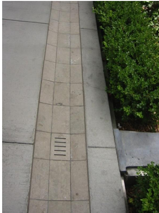
Constructed swale with drain (Credit: Stephanie Landregan)
