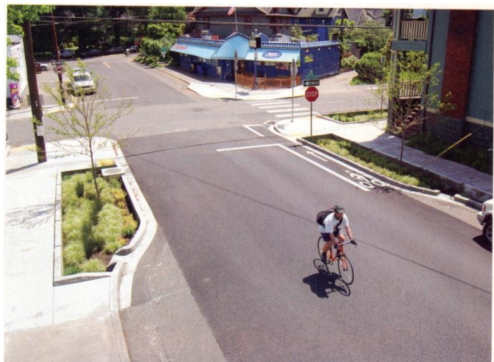
Curbside extensions with rain garden (Credit: Unknown)
