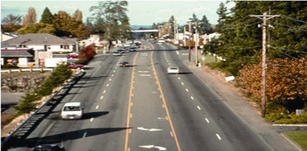
Bridgeport Way before transformation: University Place, WA (Credit: Dan Burden)
