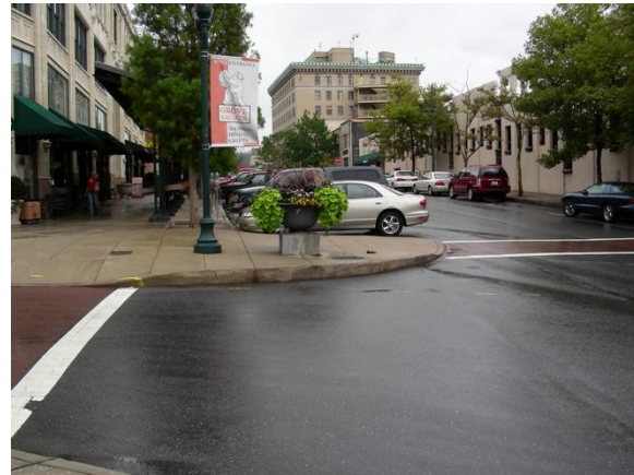
Curb extensions enhance retail districts: Asheville, North Carolina (Credit: Ryan Snyder)
