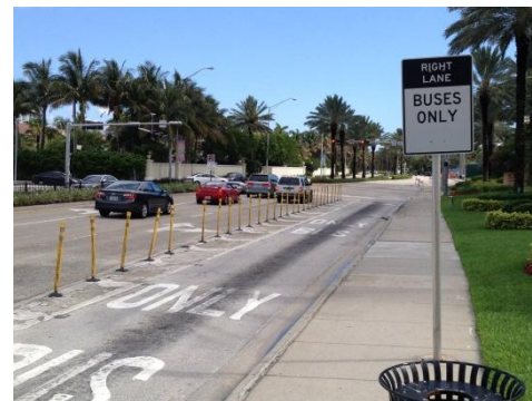
Dedicated bus lane (Credit: Kimley-Horn and Associates, Inc.)
