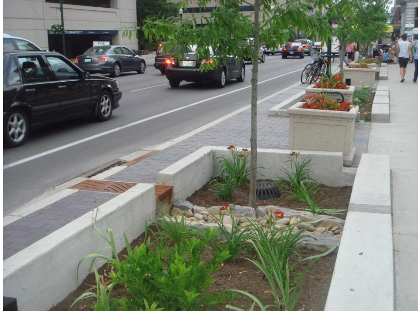
Rain garden as buffer between pedestrians and motor vehicles (Credit: Stewart Robertson)
