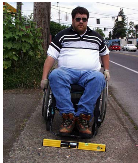
Steep cross slopes create difficulties for wheelchair users.
