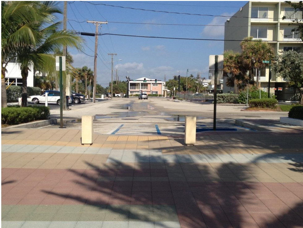
Bollards separate a street-end from the sidewalk (Credit: Kimley-Horn and Associates, Inc.)
