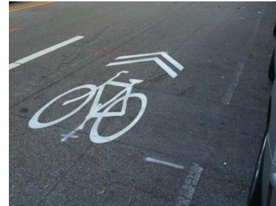
Sharrow pavement marking (Credit: Kimley-Horn and Associates, Inc.)
