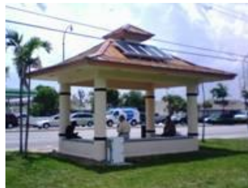
Transit shelter with solar power
