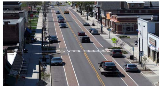
Parking assist lane (Credit: Michael Wallwork)
