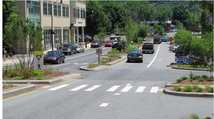
Curb extensions and medians make crossing four-lane streets safer and more manageable. Note the use of an in-street pedestrian crossing sign to alert motorists. (Credit: Dan Burden)
