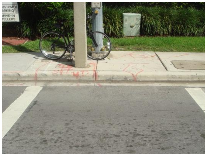
Missing curb cut ramp at crosswalk (Credit: Kimley-Horn and Associates, Inc.)
