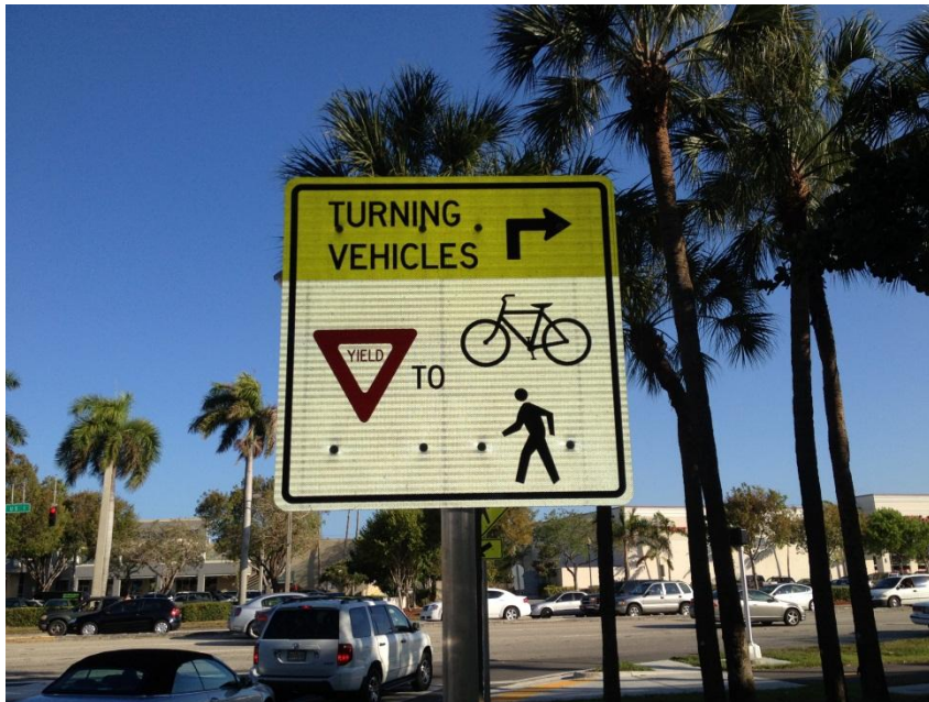
This TURNING TRAFFIC MUST YIELD TO PEDESTRIANS AND BICYCLISTS sign is an R10-15 (modified). The modification is for use on shared-use paths. (Credit: Kimley-Horn and Associates, Inc.)
