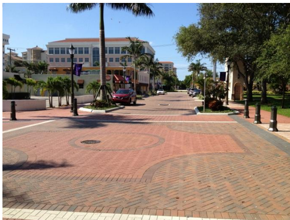
Festival street with flush sidewalks separated by bollards (Credit: Kimley-Horn and Associates, Inc.)
