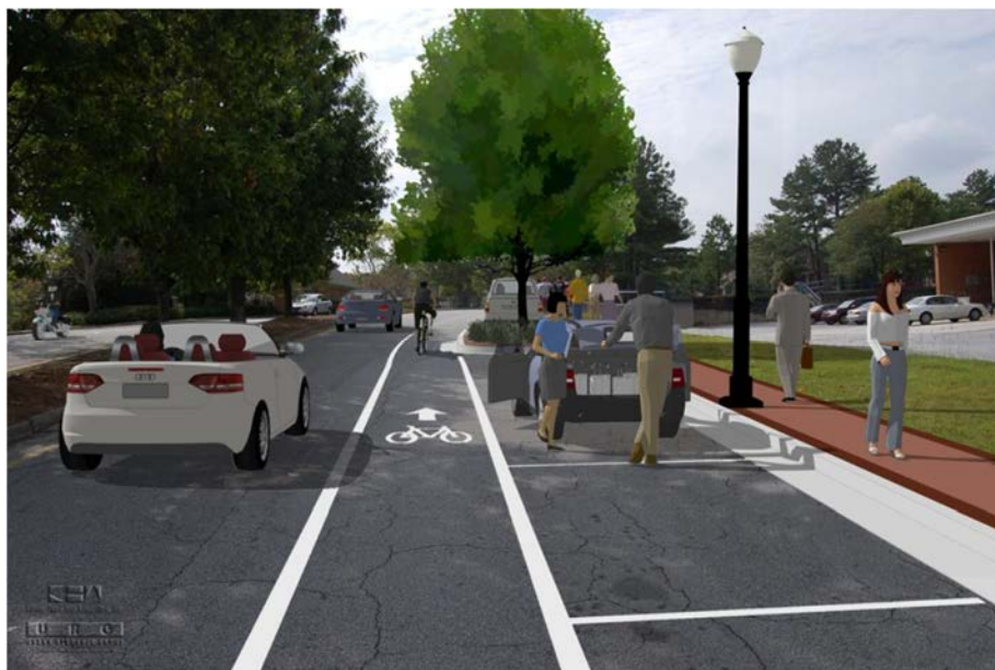
Simulation of the positive result of a 4-lane to 2-lane road diet with bike lanes and on-street parking (Credit: Kimley-Horn and Associates, Inc.)
