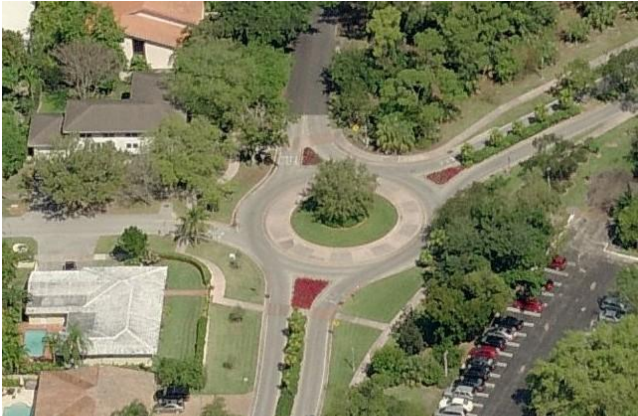
Roundabout with splitter islands for pedestrian crossings (Credit: Kimley-Horn and Associates, Inc.)
