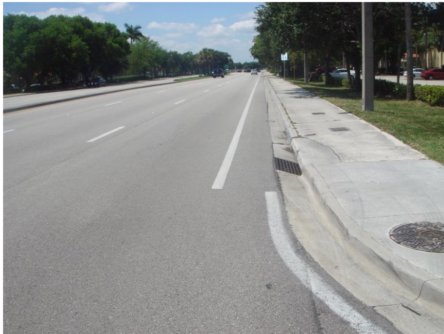
Undesignated lane. Note the corner radius striping, which allows bicycles to enter the undesignated lane.
